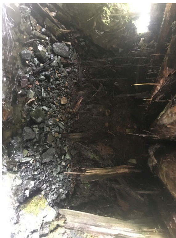
Right Bank Abutment when facing downstream
